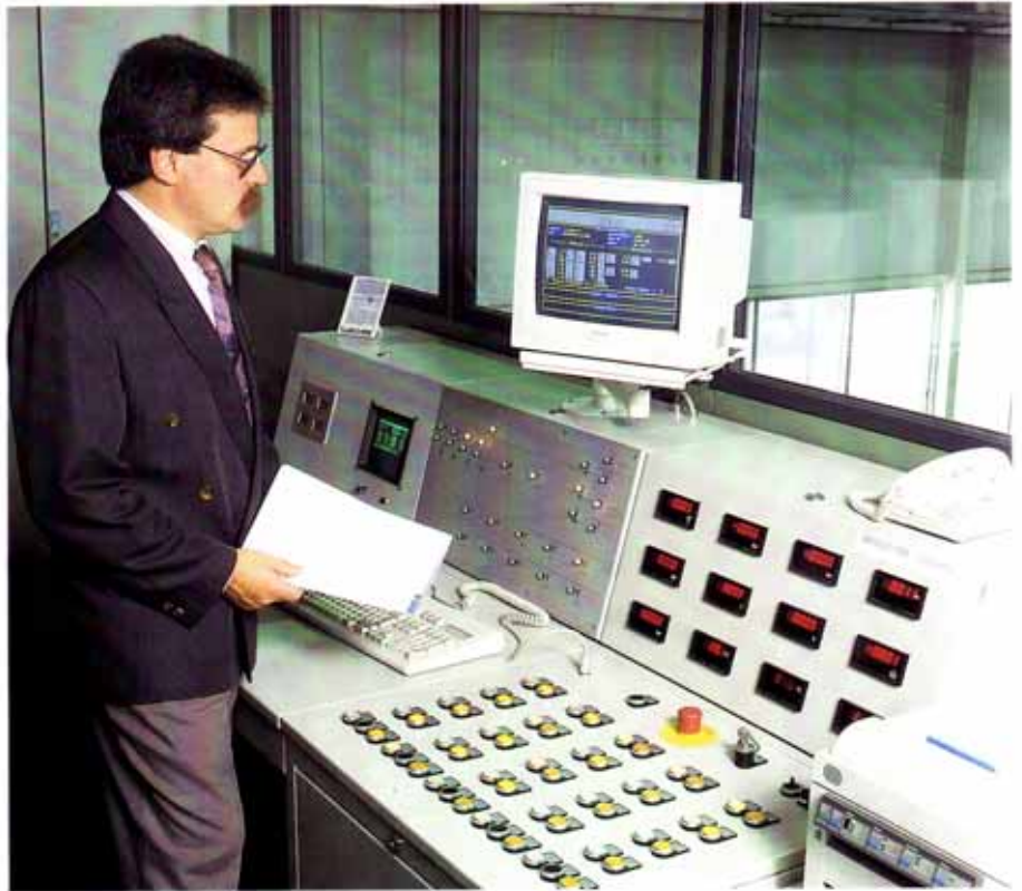
The recording, evaluation, documentation and archiving of all measured values takes place centrally via a computer at the measuring station.
