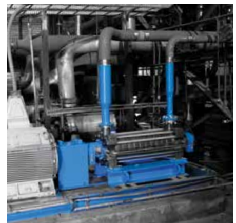
Adjustment reducers & retrofit base frame
